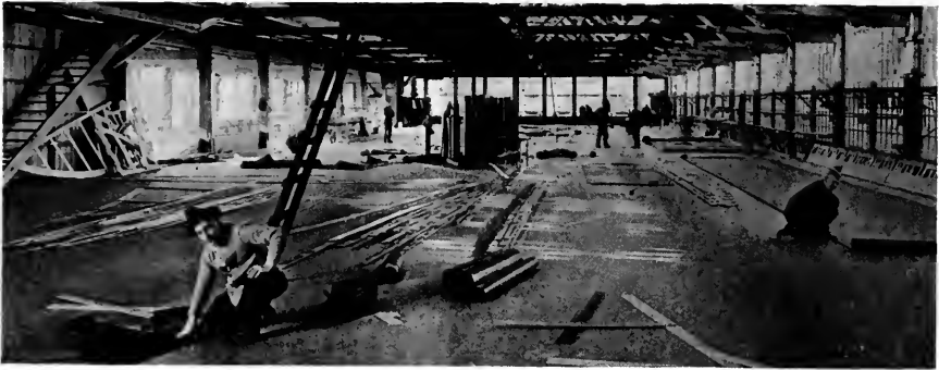
The mould loft at the Northwest Steel Company's plant furnishes ample room for laying out work.
